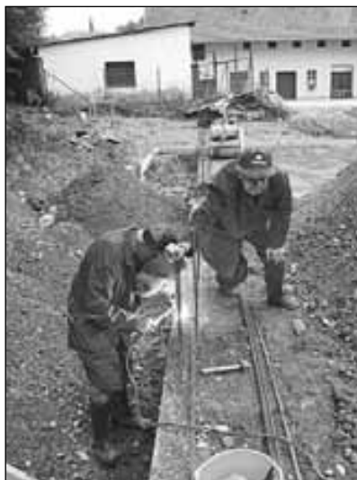
Gasilca veterana Ivan Blažič in Franc Komar varita železno armaturo
